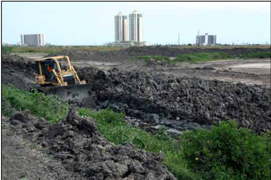
Heavy equipment operators construct dewatering ditches at the San Jacinto Placement Area as part of $1,382,700 contract to provide outflow of excess water to increase the placement area's capacity to hold more dredge material. This process is part of the district's Disposal Area Management Program which ensures placement areas are prepared for future dredging activities.
