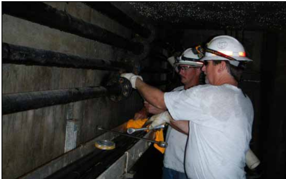
Installing the new stainless steel hydraulic pipelines are left to right, Tulsa District employees David Ford and Christopher Anderson. Crews from the Tulsa District have installed new stainless pipes in three of the districts lock and dams with two more scheduled for replacement as money becomes available. (Photo courtesy USACE employee Victor Heister)
