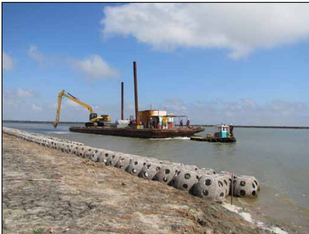
The USACE Galveston District places a final reef ball in an area that has been named the Robert Benjamin Boren Memorial Reef, located in Chocolate Bayou, Placement Area 4A. Boren, who passed away July 4, 2008, was a USACE Galveston District visionary who advocated the use of the concrete reef balls for erosion control purposes (as an effective alternative to articulated concrete block revetment systems) and to help enhance marine ecosystems. (Photo by Mike Bledsoe, USACE Galveston District.)
