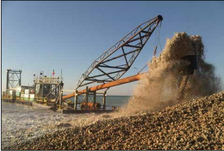
The spill barge "Shamrock" places material to construct an underwater levee that is part of a Beneficial Use Site to provide a shallow water sea grass habitat along the south side of the new channel, during the construction of the La Quinta Channel Extension Project in Nueces County, Texas. The USACE Galveston District awarded the contract in September 2011 in the amount of $33,537,027.20 to Texas-based King Fisher Marine Service LP (now known as Orion Marine Group) to complete the project by July 2013. (Photo by USACE Galveston District Civil Engineer Kenneth (Chip) Worley.)
